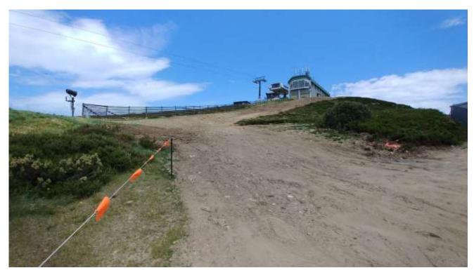
Photo 14 Haulage road that may be the source of localised sedimentation in Bogs 1 and 2.
