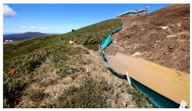
Photo 1 Source of sediment at the base of the dam embankment and upslope of Alpine Bogs.
